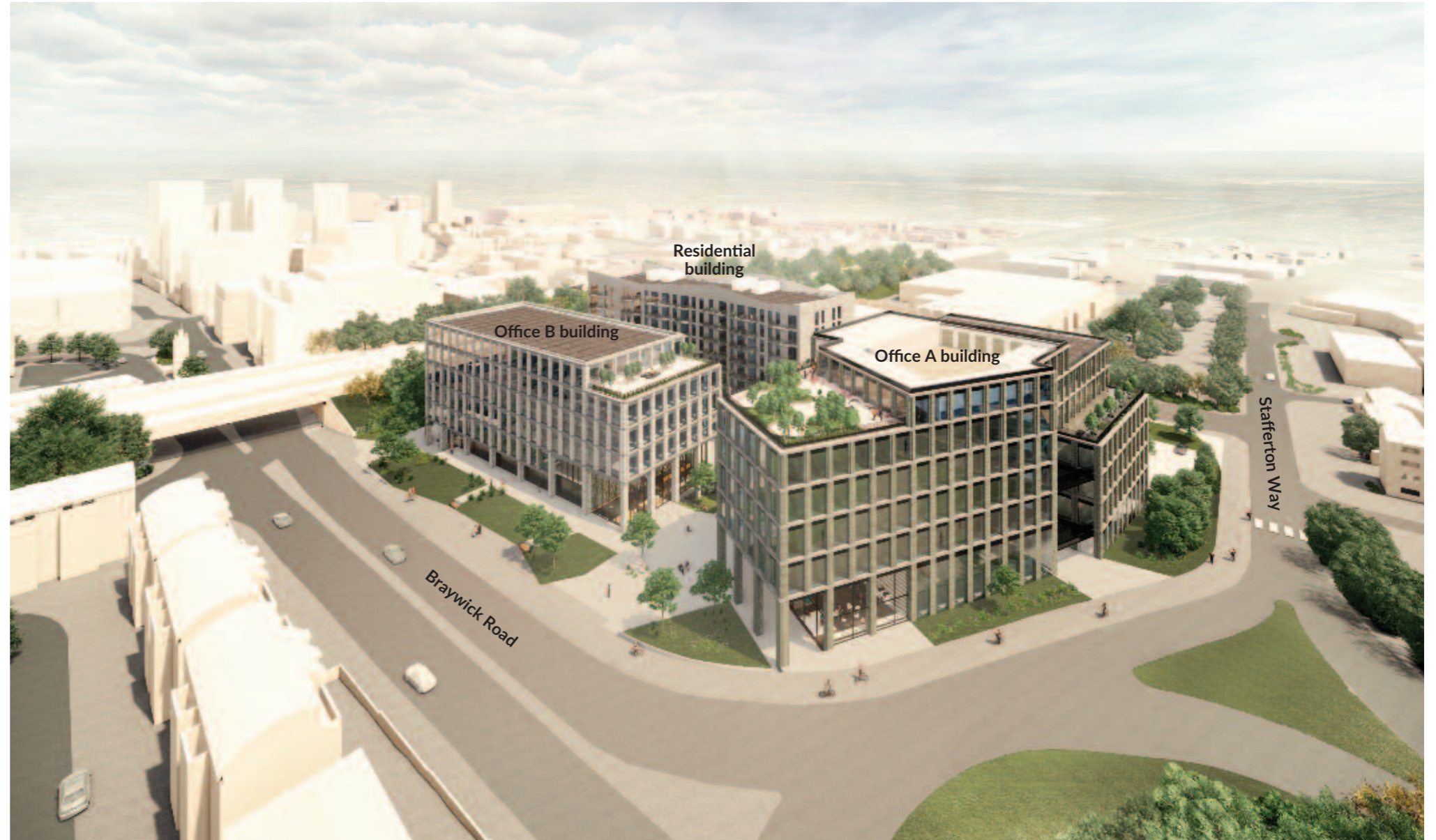
Aerial view of proposed development looking north east from Braywick Road
